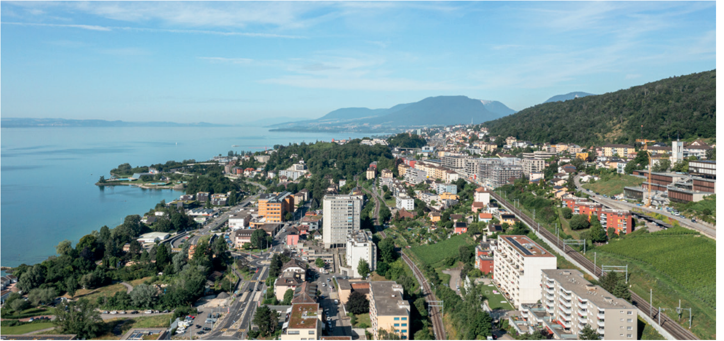
Site photo © LAST / N.Sedlatchek
